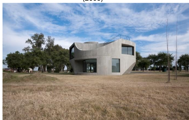
Figura 01 – Casa View, Diego Arraigada / Johnston Marklee (2009)
